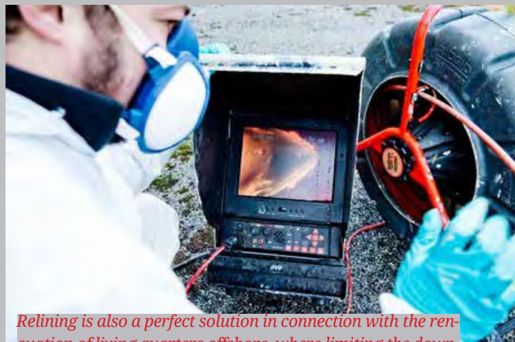
A thin layer of plastic is injected into the existing sewer pipe with a special machine. Here a renewed pipe is created that will last for 40 to 50 years. Photo: Øyvind Sætre/Aibel.
